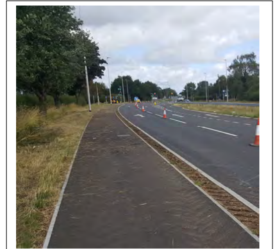
Photo 4 – Existing combined facility alongside the A449
